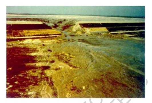
Figure 1. Failure of the Boliden lead-zinc tailings dam in 1998 (www.wise-uranium.org/mdaf.html)
