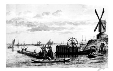
Figure 6. Mud-mills in operation. One is driven by a human treadmill, a is second driven by horsepower
