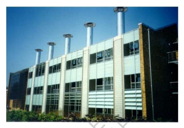
Figure 2. Modern office building with a blend of HVAC systems and classical features of natural ventilation. The BRE office building in Garston, UK uses among other features five wind towers to enhance natural ventilation.
