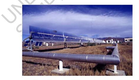
Figure 1. Medium concentration solar collector. One-axis parabolic trough collector (PSA, Spain)
