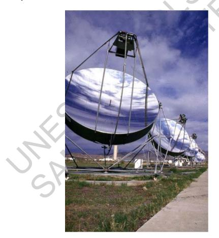
Figure 2. High concentration solar collector. Parabolic dish solar reactor (PSA, Spain)
