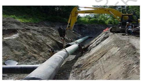
Figure 2. Open cut installation of buried pipelines.
