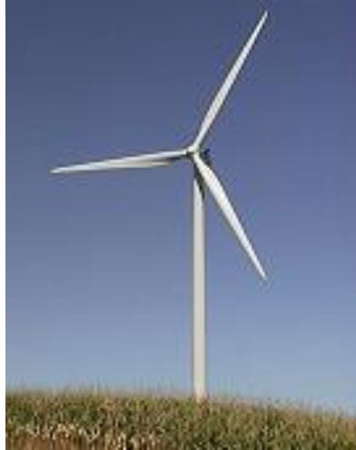
Photo 1. Wind turbine tower
