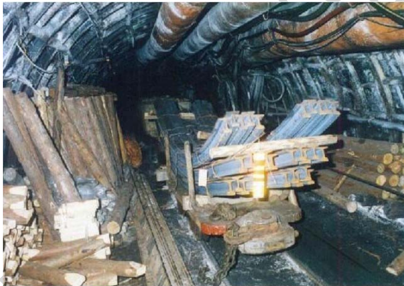
Figure 4: Material transport by a rail-mounted system
