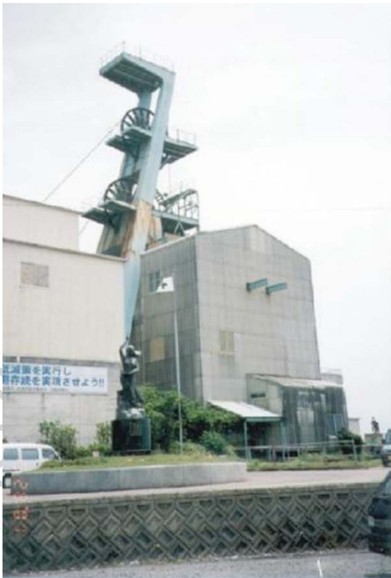
Figure 1: Vertical shaft at Ikeshima Colliery
