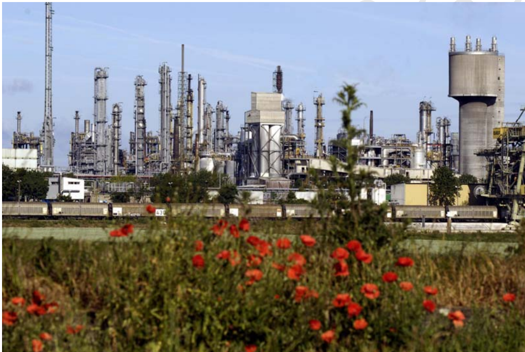
Figure 1. A reactor for steam cracking (breaking the molecules of heavier hydrocarbons into smaller ones) occupies central part of a plant in BASF, Ludwigshafen, Germany (copyright BASF).
