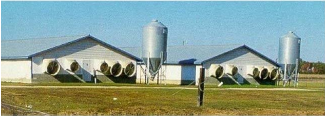
Figure 3. An example of ventilation fans in a swine facility. Fans for each building have a ventilation capacity of approximately 50 \text{ m}^3 \text{ h}^{-1} .
